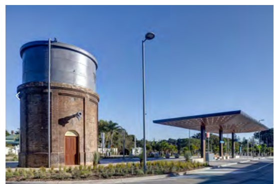
Byron Bay Bus Interchange
